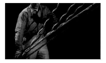
2.04 Align the crossovers marks and make one or two wraps of the upper section. Next, do the same with the lower section. Then apply each section alternately, one wrap at a time, until the second leg is applied for two-thirds of its length.
