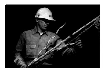
2.05 Now complete the application of the deadend one section at time, applying the short leg first. (This method allows the ends to be snapped into place more easily.)
