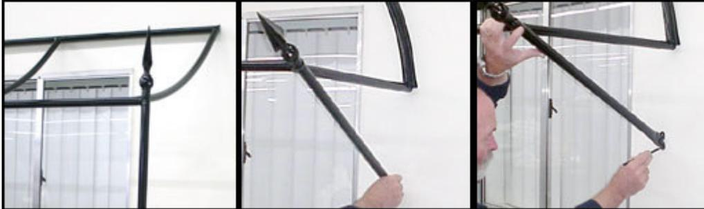
9. Remove the frame. Drill holes in the mounting surface for the Support Arm Camel Back Hinges, and then securely fasten to the wall. (NOTE: Use the appropriate caulking of the fasteners to prevent leakage.)
