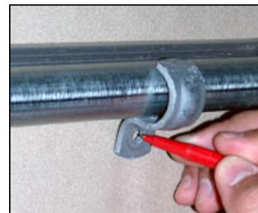
3. Remove the Head Bar, and then drill pilot and/or anchor holes for mounting the J-Clips. *(NOTE: With varying building construction, mounting anchor fasteners are NOT included. We recommend consulting with a contractor or local hardware store for the best mounting anchor solutions.)*
