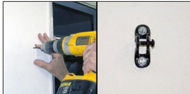
10. With the frame level, centered and the angle is positioned correctly, use a rubber or rawhide mallet to strike the J-Clips firmly into place. Tighten ALL J-Clip anchor bolts to the wall. (NOTE: Use the appropriate caulking of the fasteners to prevent leakage. The J-Clips are pressure-fitted and hammering may or may not be required.)
