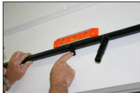
2. Determine and mark the mounting points for the J-Clips on the underside of the awning. (*NOTE: We recommend mounting one J-Clip two inches inward from the frame ends, then equally spaced in between.*)
