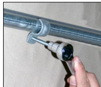
7. Place the top frame on the loosely mounted J-Clips and hold against the wall in the required location. Level, center and adjust the Head Bar positioning, if necessary. *(NOTE: A second person may be needed to hold the frame.)*
