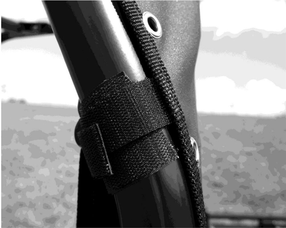
5. Once the door is hung by the double-sided Velcro strips finish off the edges by matching up the 4" adhesive strips with the Tabs sewn to the edges as seen in the photos below.
