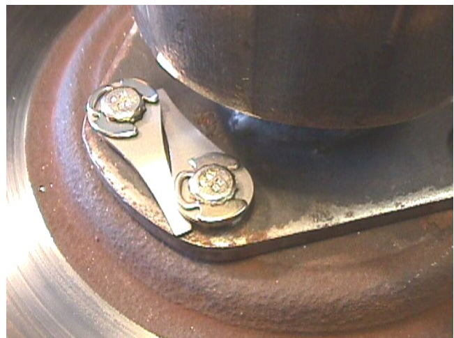
Picture 10 – Clips installed
