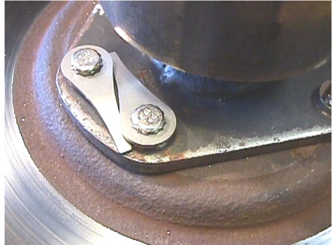
Picture 8 – Installing the tabs
